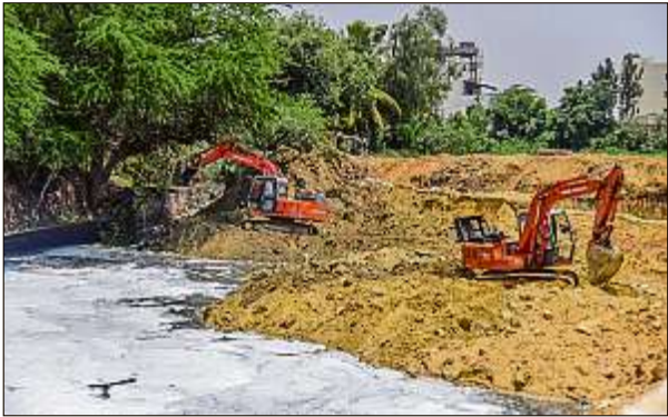
Authorities expect to exhume 6.60 million cubic metres of silt from Bellandur Lake. The silt could be used in 15,000 acres of farmland. DH PHOTO
